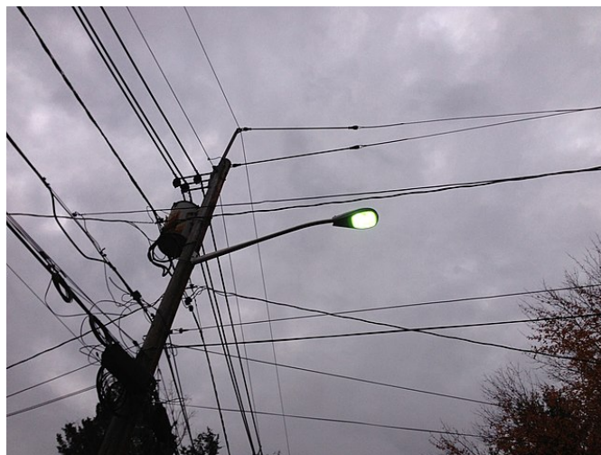
Figure 7 Mercury vapour street light Ewing, New Jersey.
